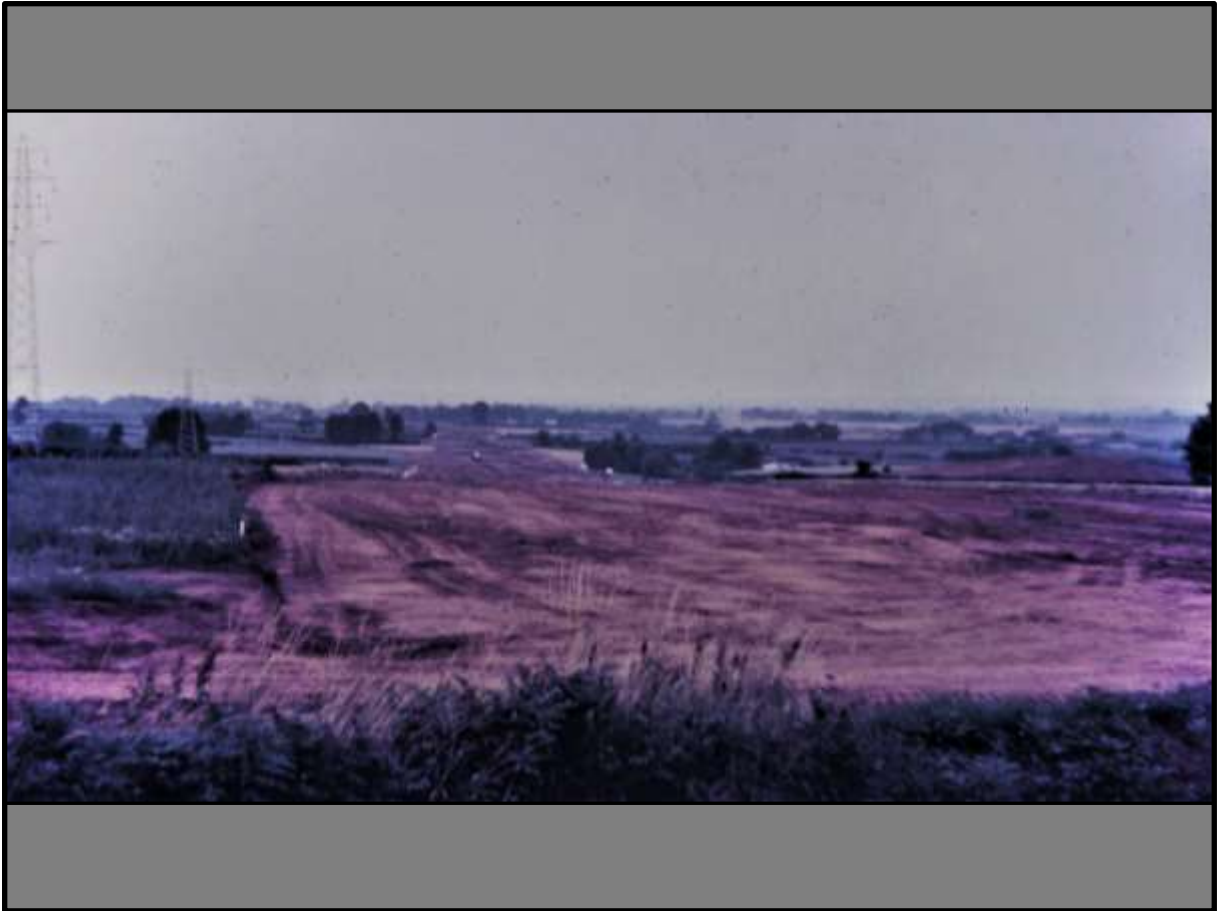
The start of work looking north from Moon Lane, nr North Newton.
