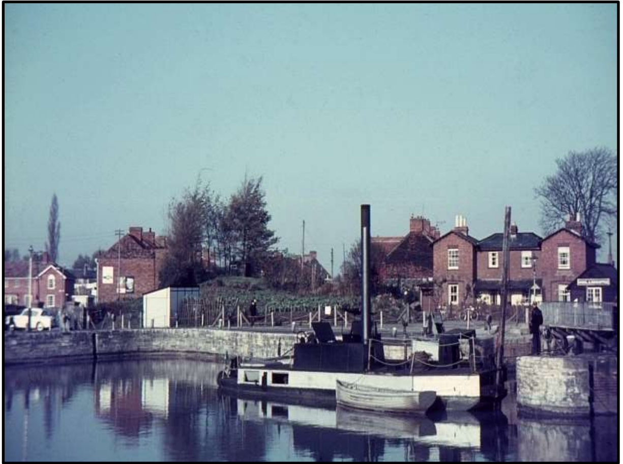
The drag boat, unofficially known as “Bertha”, built in Bristol. She worked by dragging herself back and forward across the dock on fixed chains and pulling a scraper blade which pulled accumulated silt to a position that could be flushed out into the river through culverts in the dock floor.
